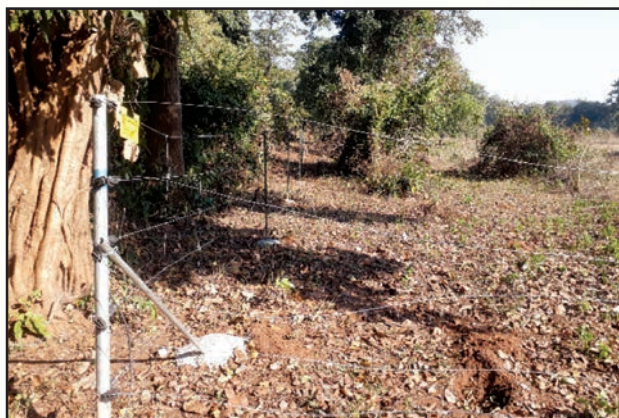
Photo-voltaic (solar) fencing, Nunvet
