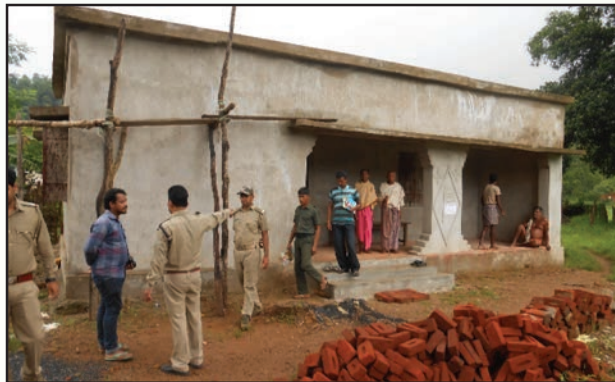
The Anganwadi under construction
