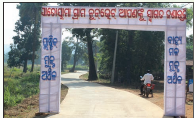
The New Concrete road, Nunvet
