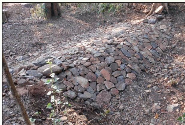
The Nalas Treated with LBDC structures, Nunvet
