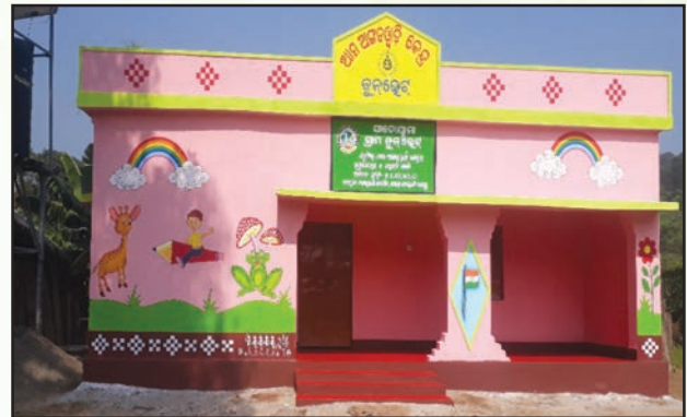
The Completed Anganwadi
