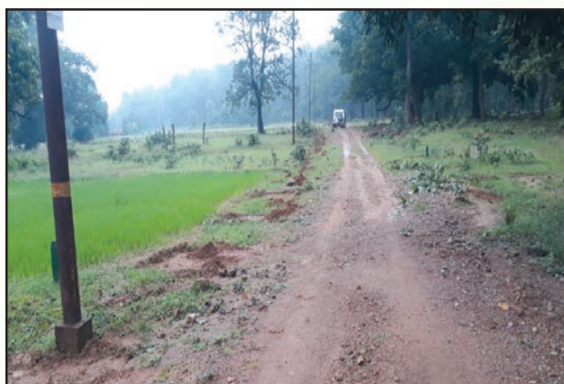
Pitting work done by the villagers
