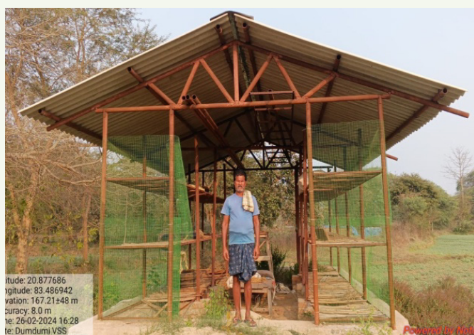
Construction work of storage structure is under progress
