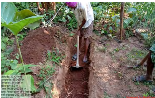
Renovation of staggered trench at Bijamal VSS, Bolangir Forest Division
