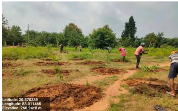
Soil working in ANR With Gap Site at Muribahal, Bolangir Division
