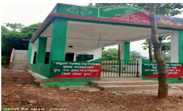
VSS Building-cum-IGA Facilitation centre of Gujahuli VSS of Deogarh Division
