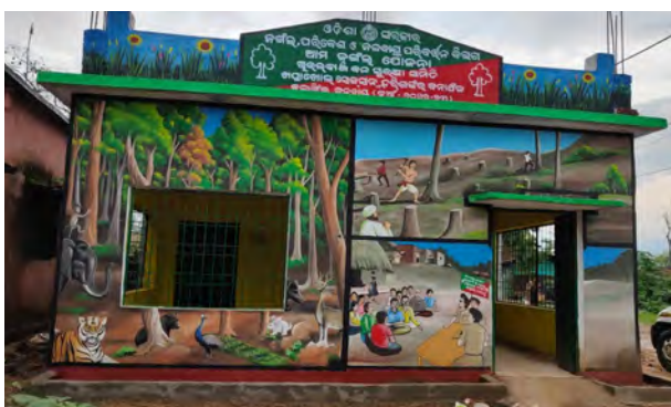
VSS Building at Chaulbanji VSS, Harishankar Range of Bolangir Division
