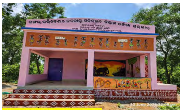
VSS Building at Ambatumba VSS of Jaleswar Range, Balasore(WL) Division
