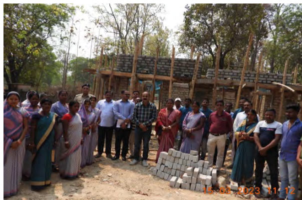
Review of VSS building-cum-IGA Facilitation Centre at Bhalughara VSS, Keonjhar Division
