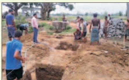
Construction work of the VSS Building
